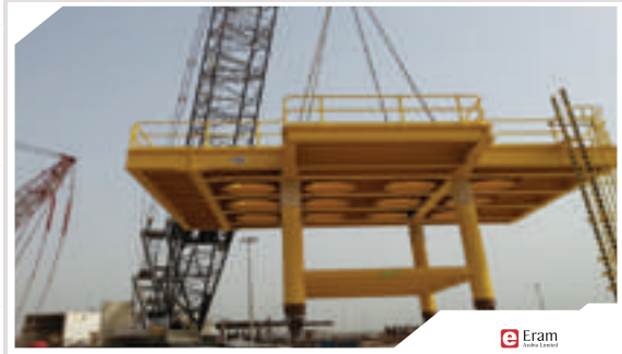
Zulf 510 Drill Deck
