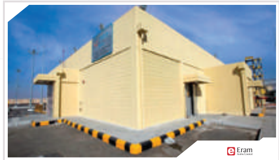
Civil & Asphalt Works @ SVC Al-Jouf-2
