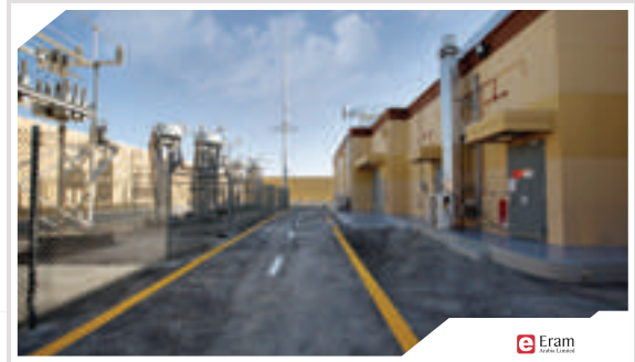
Construction of Al Salmaniyah
