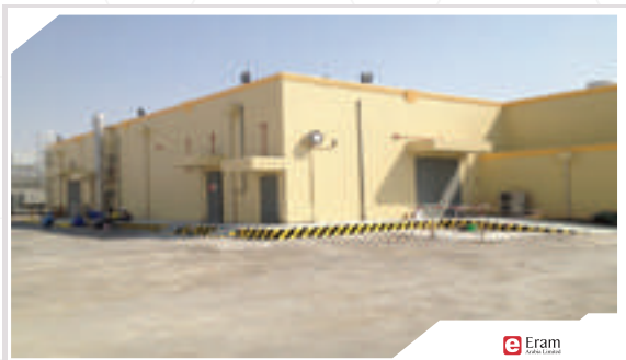
Construction of Ghassaniyah/ Al Hassa
